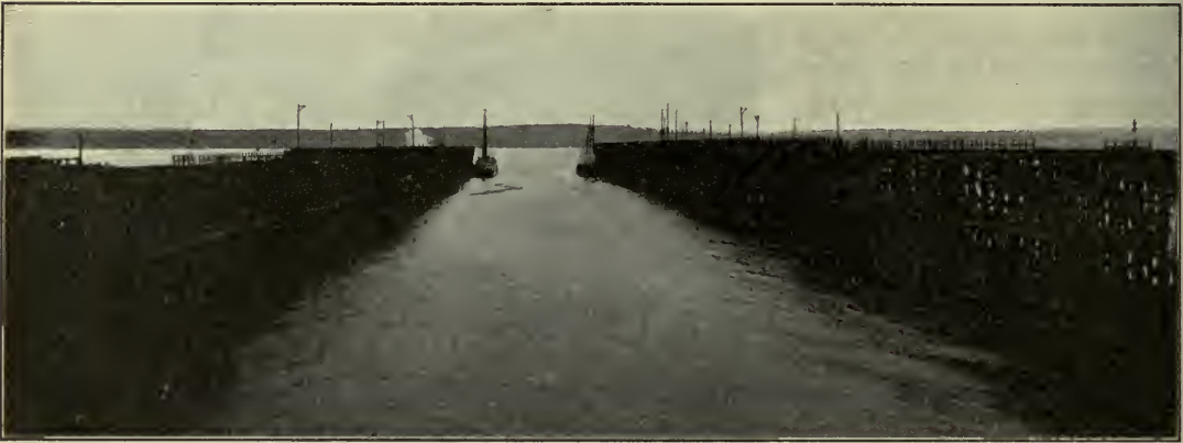
FIG. 253.—The great ore docks on the shores of Lake Superior. Trains loaded with ore run out onto these docks and dump their ore into large bins, from which vessels are loaded.
